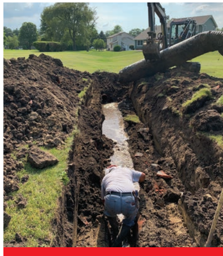
Fratco drainage installation at Tippecanoe Country Club.
